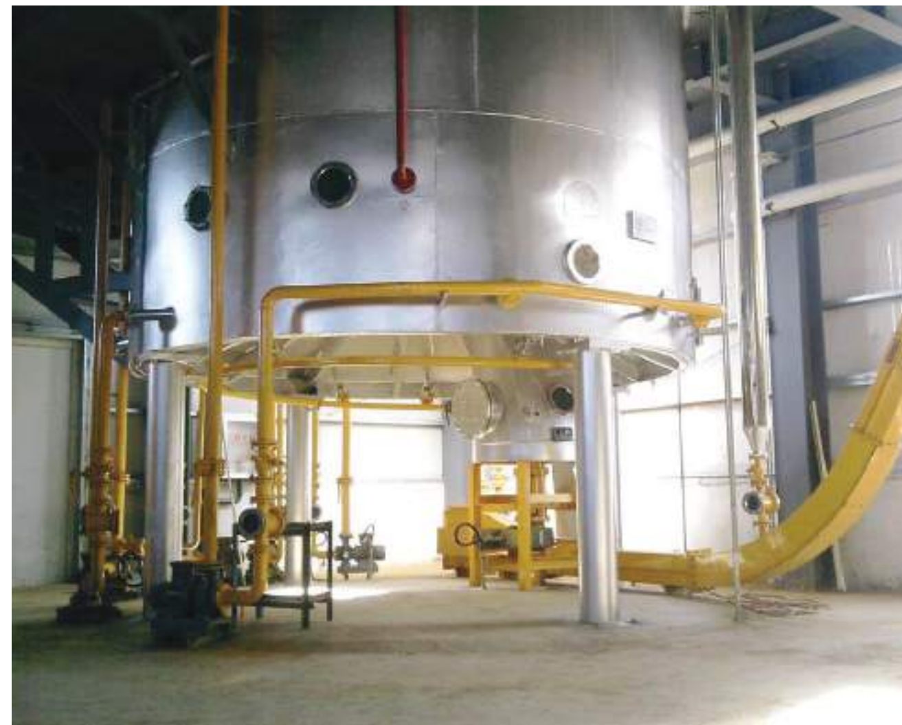
Pyrethrum Processing Factory
